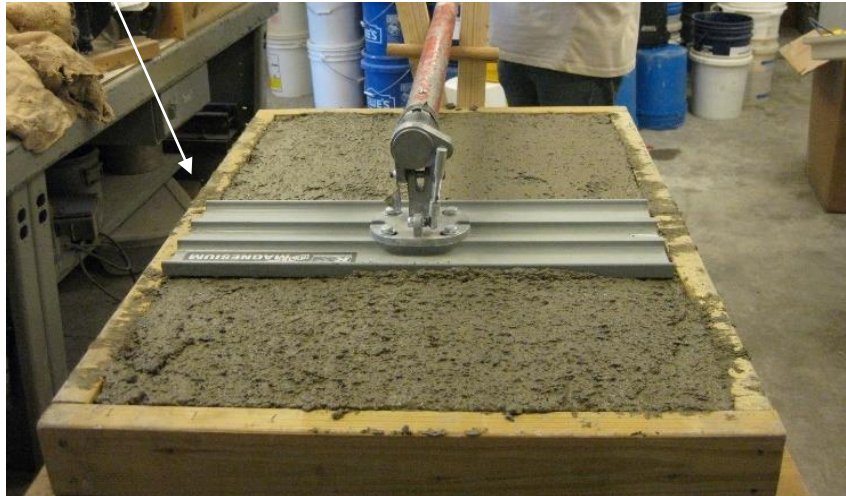
First Pass with Bull Float
