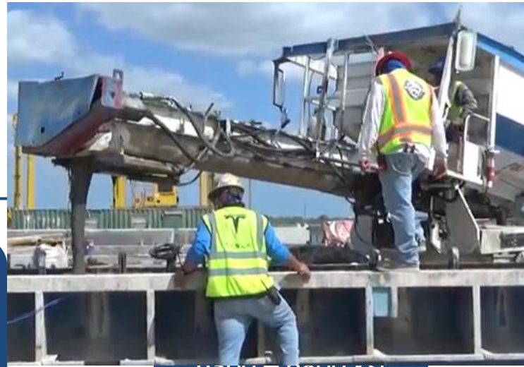
Fabrication of UHPC Girder Specimen
