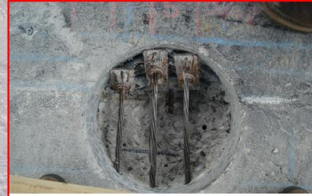
**Severed Anchors by Core Drilling**
