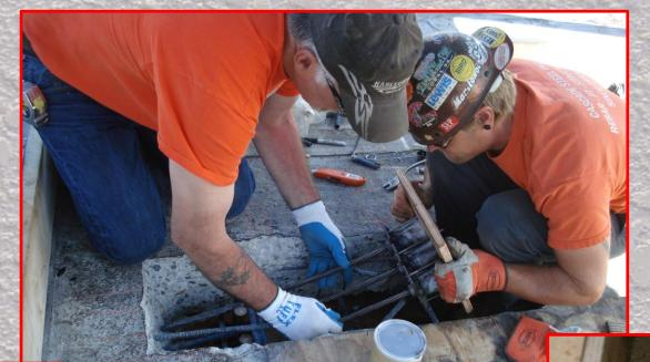
**Installing New Anchors**
