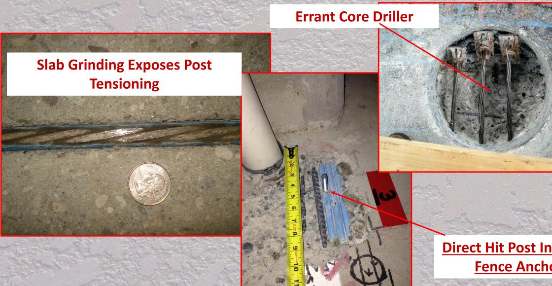
**Direct Hit Post Installed Fence Anchor**
