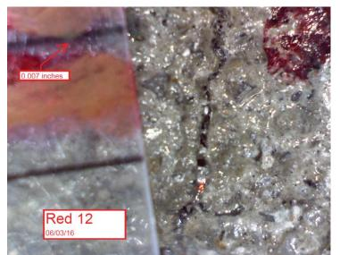
Crack #12 on three separate dates to confirm stability.
