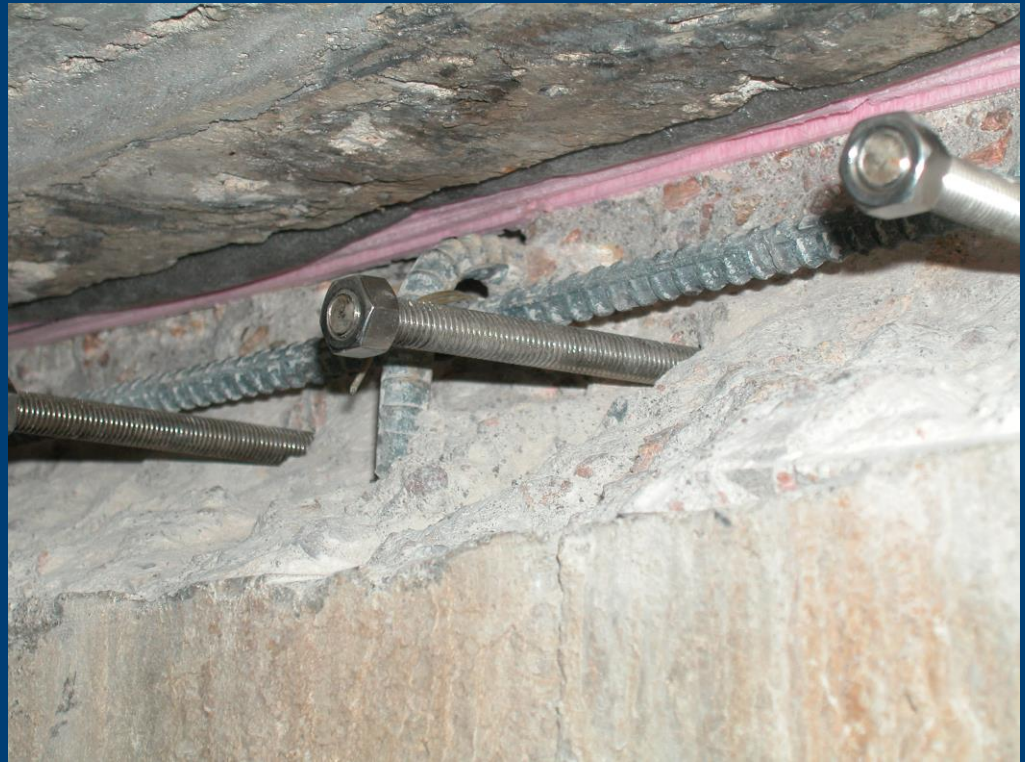
Support for P.T. slab repaired
