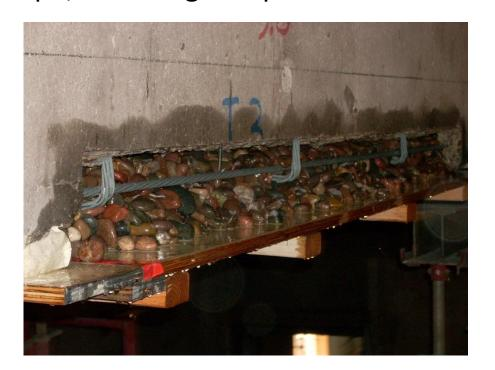
Do not use caulk. Caulk can yield under the head pressure from the grout.
