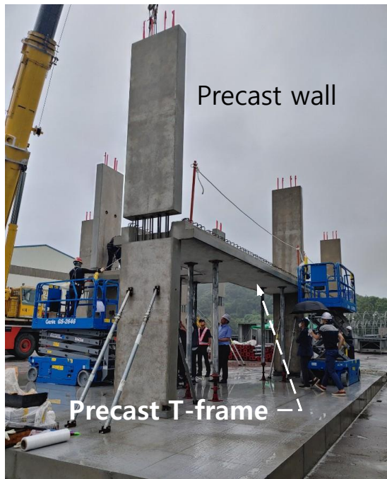
(a) T-frame floor for underground parking lot in apartment buildings
