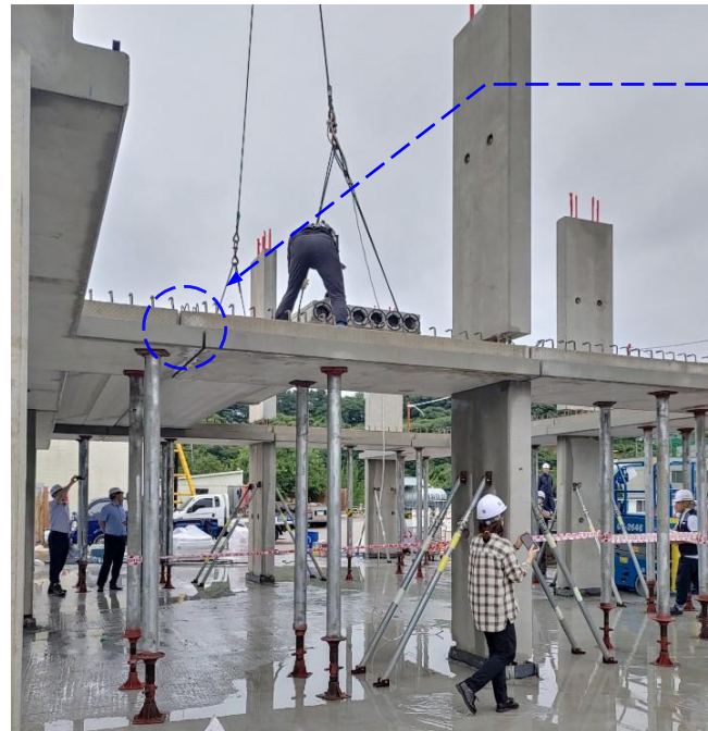
(a) T-frame floor for underground parking lot in apartment buildings
