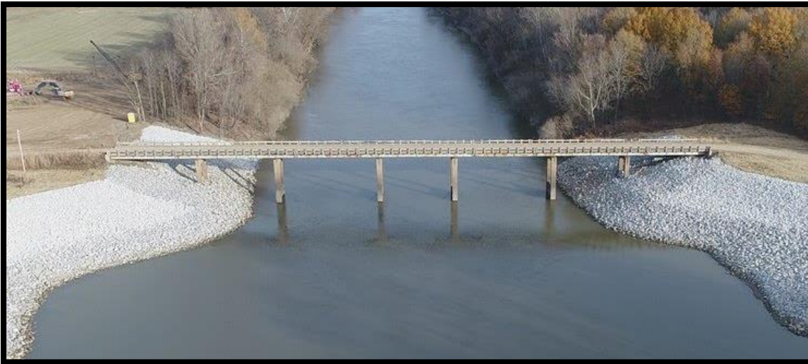
Resiliency in Retrofit of Existing Structures
