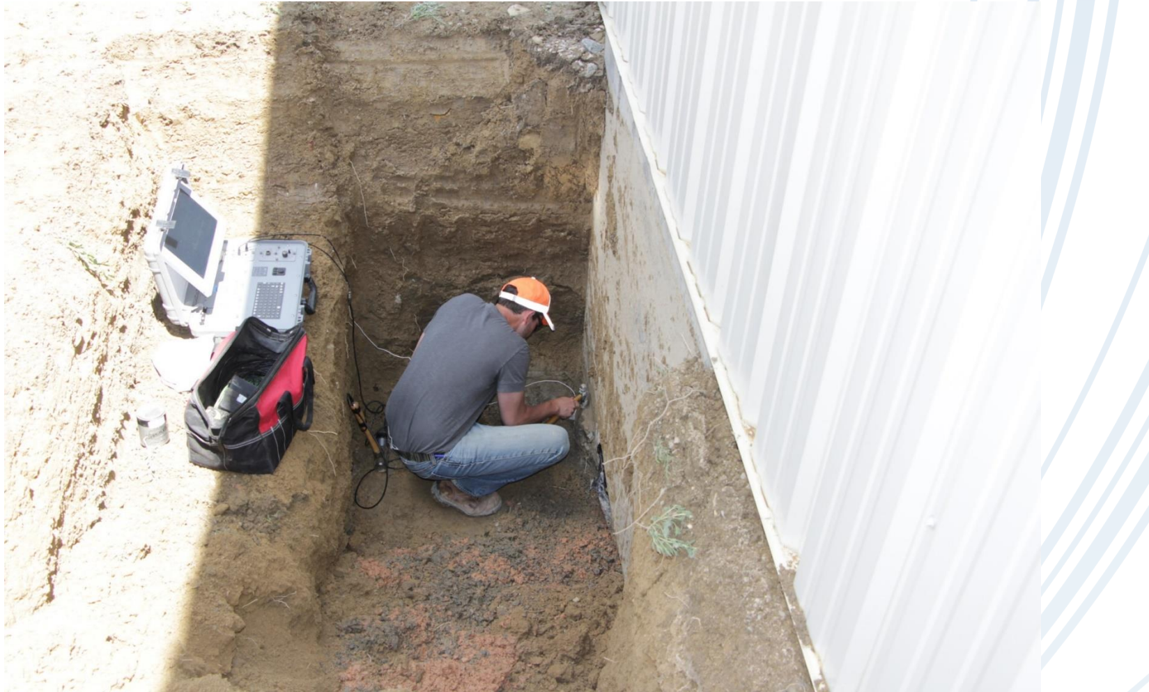
SE Test being Performed on a Drilled Pier
