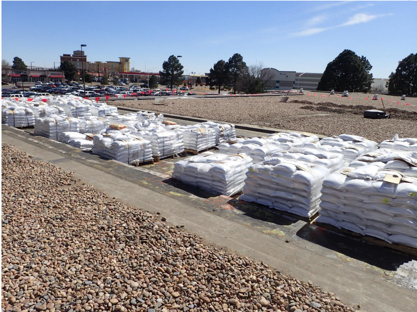
Load Testing in Progress
