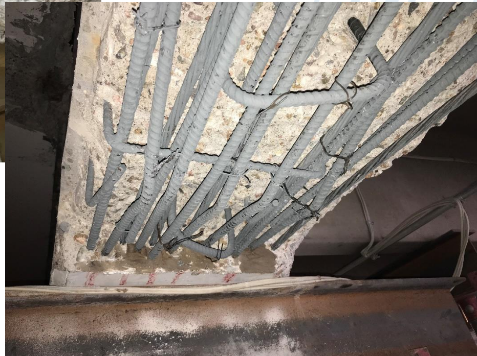
Reinforcing before and after repair Supplemental reinforcing added
