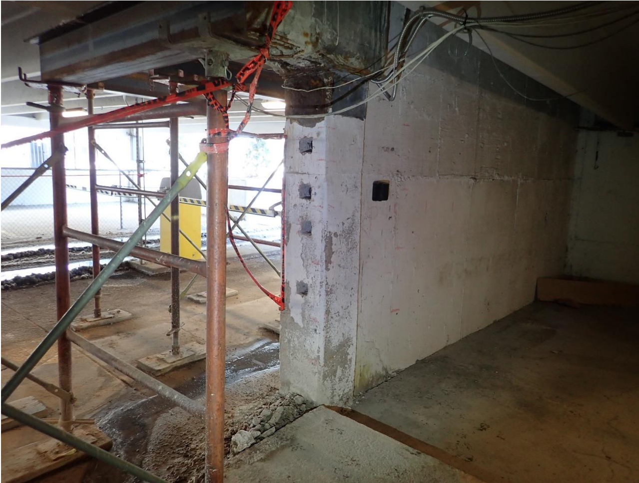
Dowels were installed with the structure shored
