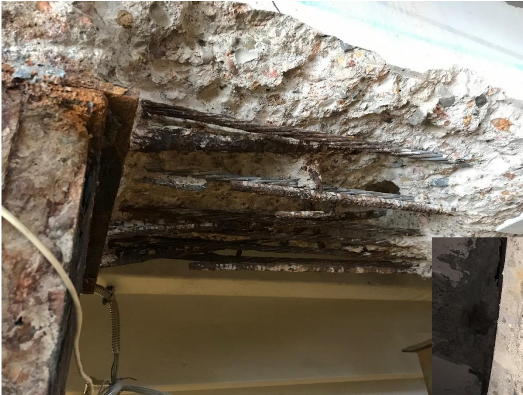
Reinforcing before and after repair Supplemental reinforcing added
