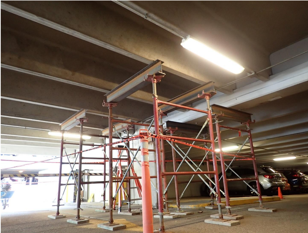
Shoring for Double-Tees and Ell Beam to Slab-on-Grade
