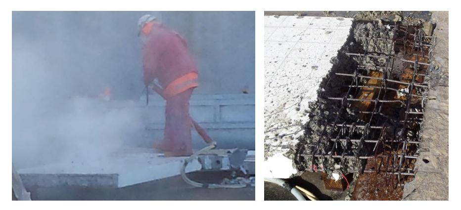
Removal of Concrete (Hydro-demolition)
