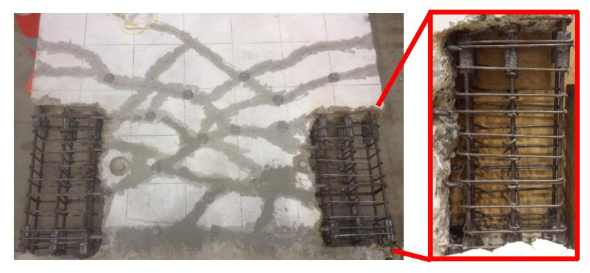
Reinstatement of reinforcement & Preparation for crack injection
