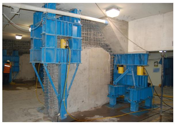
Repair of RC wall in 11-story building in Vina del Mar after Maule, Chile (2010) Earthquake (photo courtesy of Jorge Carvallo) Repair of RC wall in 18-story building in Santiago after Maule, Chile (2010) Earthquake (Sherstobitoff et al, 2012)
