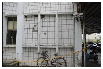
Infill Material Assumed to be Hollow Clay Tile (HTC)
