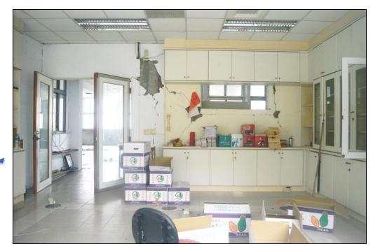
Kitchen items remained largely in place in spite of damage to the surrounding structural elements.
