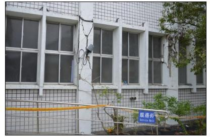
Vertical & Diagonal Cracking at Columns A7 & A8
