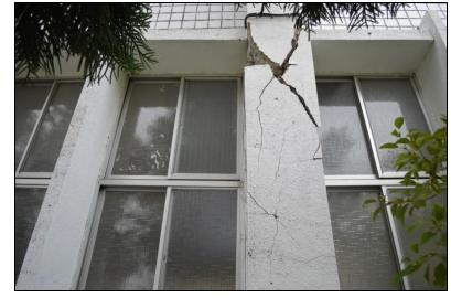
Diagonal Cracking at Column A9
