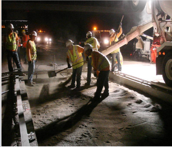
Placement of Bedding Material
