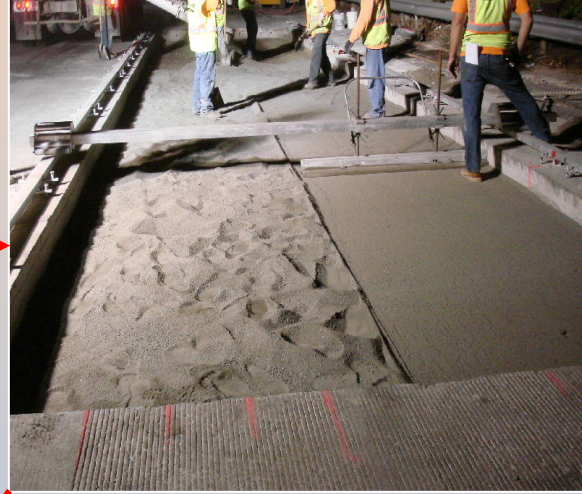
First Grading Pass
