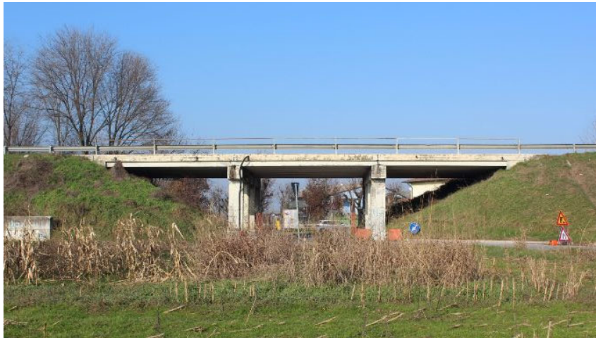
SMALL ROAD BRIDGE SOUTH BRESCIA (IT)
