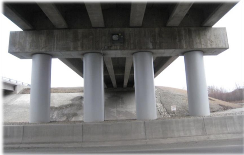
O'Malley Bridge (Courtesy, AKDOT)
