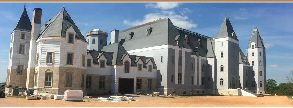
Category: Contractor: Location: Application: Helix Dosage: Residential Huff Construction Highlandville, Missouri Walls, Slabs, Precast Trim and Cladding Walls - 22.5 - 45 lbs/yd, (27 kg/m<sup>3</sup>) Slabs - 34 1bs/yd (20 kg/m<sup>3</sup>) Roof - 60 lbs/yd (36 kg/m<sup>3</sup>) Cladding - up to 140/lbs/yd<sup>3</sup> (85 kg/m<sup>3</sup>)
