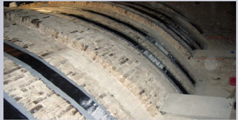
Reinforced barrel vault
