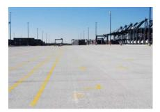
Surface After Grinding (¼ inch Under 10 ft Straight Edge)
