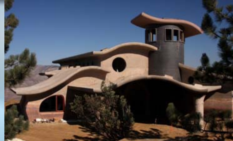
A house that is all Type K Concrete. All roofs are monolithic concrete without roofing. The entire structure has only one joint
