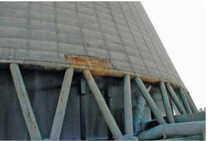
A project on determining the extent of degradation and the structural bearing capacity margin in severely damaged cooling towers is being performed at EPRI.
