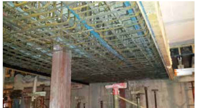
Post-tensioned drop panels with formwork
