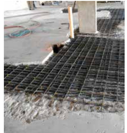
Fourth-level transfer slab crack repair after demolition
