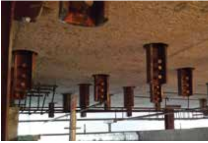
Steel lug keys and reinforcing bars in the drop panels
