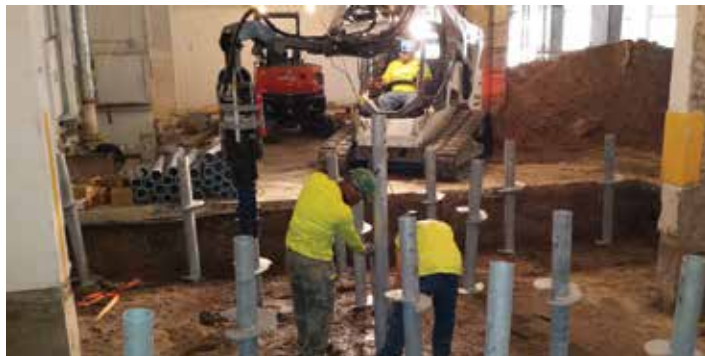
Helical pile installation in the foundation area
