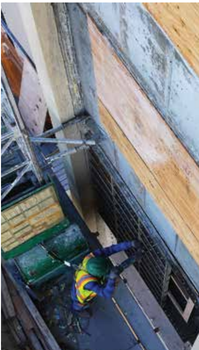
Exterior shear walls
