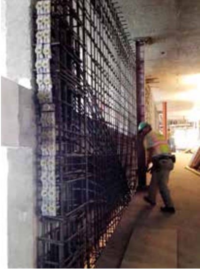
Steel and cables in the post-tensioned beam
