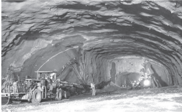
Fig. 1.1a—Typical heading: large tunnel with drill rig.
