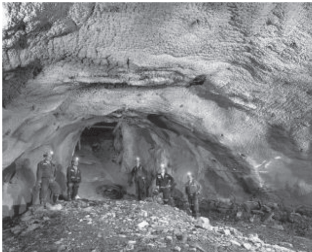
Fig. 1.1c—Typical heading: mine.
