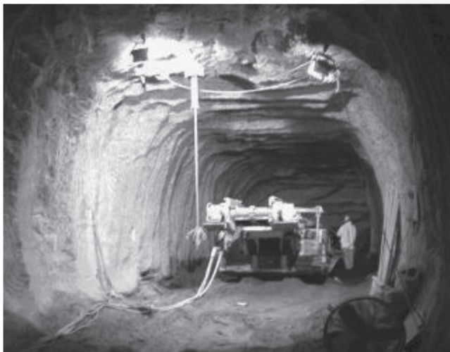
Fig. 1.1b—Typical heading: small tunnel with drill jumbo.
