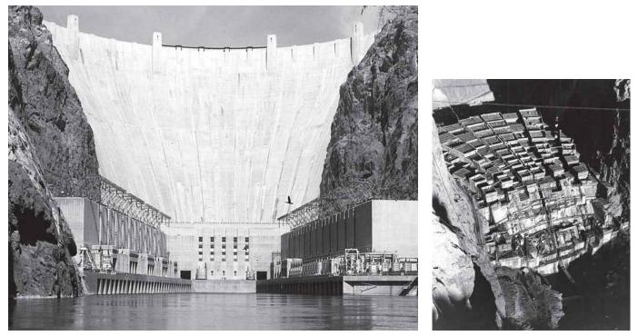
Hoover Dam was the first modern mega project—the greatest dam constructed in its day. For nearly two years, every day, around the clock, a bucket of concrete was dumped into a form every 60 seconds. The dam was raised to 726 ft (221 m) by placing and cooling concrete in 230 massive blocks (December 1933 photo). *Photo courtesy of the U. S. Bureau of Reclamation.*
