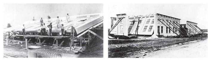
One of the earliest site-cast, tilt-up wall panel construction projects was undertaken circa 1907 by Robert Aiken at Camp Perry, OH. The wall was cast upon a large tipping table (left). After 48 h, when the concrete was solid, jacks tipped the wall into position, the wall was braced, and the platform moved to the next position.
