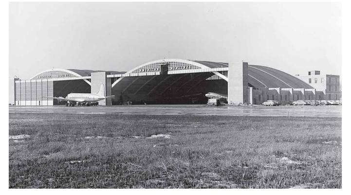
The reinforced concrete thin shell American Airlines hangar at Chicago's Midway Airport, built in 1947-1948, was one of the largest commercial airline hangars at the time; eight DC3s could be serviced in each hangar at one time. Each hangar had a clear span of 257 ft (78 m) with a rise of 42 ft (13 m). *ACI archives. Photo courtesy of Ammann and Whitney.*
