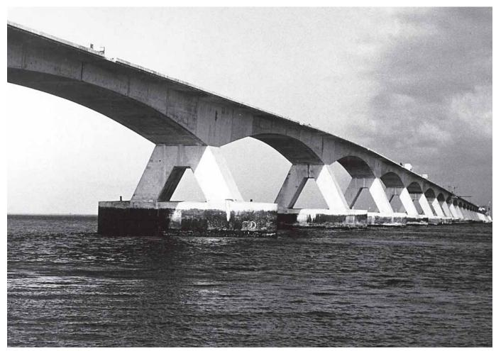
The mid-1960s saw completion of the Oosterschelde Bridge in the Netherlands, the longest bridge in Europe at the time. The 3 mile (4.8 km) bridge featured a precast, prestressed continuous hollow box structure supported on 54 mammoth piers. *ACI archives. Photo courtesy of Netherlands Consulate General Commercial Division.*
