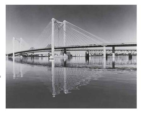
The first cable-stayed bridge with a concrete superstructure to be built in the U.S. was the Pasco-Kennewick Intercity Bridge crossing the Columbia River in Washington state, which opened to traffic in 1978. The main spans were 407 ft (124 m), 981 ft (299 m), and 407 ft (124 m). The bridge girder, structurally continuous along its entire length, was assembled from large precast prestressed concrete elements.
