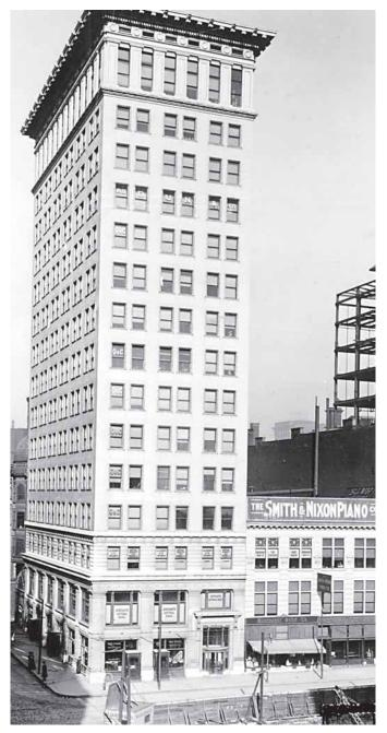
The first reinforced concrete skyscraper in the world, the 16-story, 210 ft (64 m) high Ingalls Building in Cincinnati, OH, was built in 1902-03. Up until that time, no building more than two stories high had been constructed in reinforced concrete. Henry N. Hooper, the structural engineer, prepared the design using the Ransome system of reinforced concrete. (This photograph was taken in 1906.)
