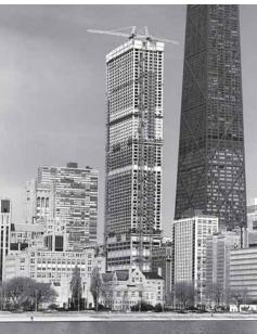
Water Tower Place, Chicago, a 75-story reinforced concrete building was higher than any reinforced concrete building when it was built in 1972-1975. The 859 ft (242 m) tall building featured a concept combining tubular design for the upper 63 stories with conventional design for the lower 13. Column concrete strengths varied from 9000 to 4000 psi (62 to 28 MPa). Lightweight aggregate concrete was used in all floor slabs.
