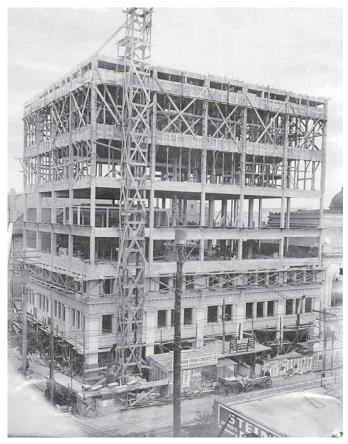
The YMCA Building in Jacksonville, FL, built in 1908-09, was said to be Florida's first large reinforced concrete frame structure. It featured a running track suspended over the gymnasium by cantilevered concrete beams. Architect: H. J. Klutho. Builder: Southern Ferro Concrete Co.
