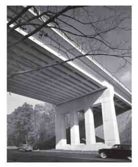
Walnut Lane Bridge, built in 1950 in Philadelphia, PA, was the first major prestressed concrete bridge in the U.S. The bridge's 13 parallel 160 ft (49 m) long main span girders were also the longest prestressed girders in the U.S. for a number of years. *Photo courtesy of the Portland Cement Association.*
