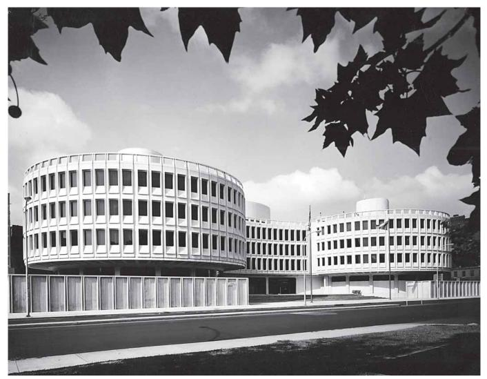
The only cast-in-place concrete above the foundation in the Philadelphia Police Administration Building was the elevator-staircase core. The rest of the superstructure was precast and prestressed. *Photo courtesy of the Portland Cement Association.*
