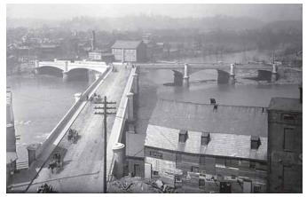
The concrete Y Bridge in Zanesville, OH, was completed in 1902 when use of concrete was still relatively novel in the midwest. The bridge's peculiar shape stemmed from the nearly right-angle convergence of the Muskingum and Licking Rivers near the city center. The bridge, with a combined length in its three branches of 970 ft (295 m), featured extremely flat arch spans. *Photo courtesy of Ohio Historical Society.*
