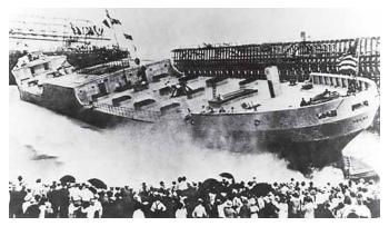
The concrete ship U.S.S. Selma was launched in June 1919. It was the first large vessel to be launched sideways. The tanker had a length of 434 ft (132 m), a beam of 43 ft (13 m), and a draft with full cargo of 26 ft (8 m). The ship's reinforced expanded shale lightweight concrete hull had a thickness of 5 in. (130 mm) on the bottom and 4 in. (100 mm) on the side. *Photo courtesy of Expanded Shale, Clay, and Slate Institute.*
