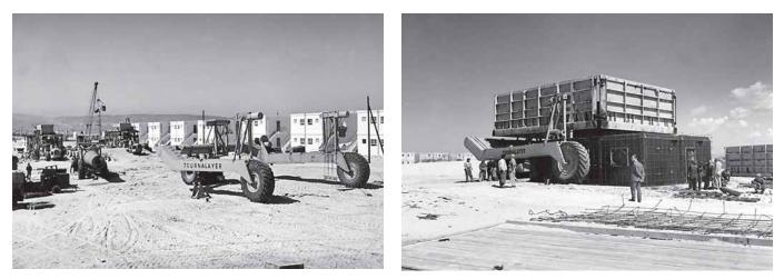
Thomas A. Edison developed a mass production system of building concrete houses in one-piece metal molds circa 1910. R. G. LeTourneau took the method to new heights in the 1940-1950 decade. One of the most notable attempts at large-scale concrete prefabrication of homes was the LeTourneau process invented in 1946. The house-molding machine was used to build a neighborhood in Longview, TX, in the late 1940s and later in Haifa, Israel, in the 1950s.
