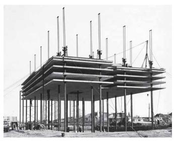
The lift-slab method of construction featured roof and floor slabs that were cast on a base slab with a separating membrane between slabs. Powerful jacks seated on columns raised the slabs to their final position where structural connections between slabs and columns were made.
