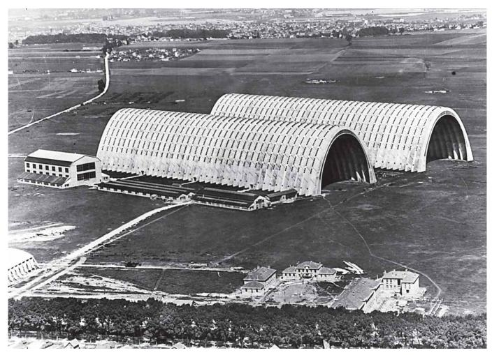
One of the earliest applications of mechanical vibration in placing concrete was that used in building the dirigible hangars at Orly, France, 1921-1924. Utilizing a system of corrugated arches—40 corrugations 10 to 18 ft (3 to 6 m) deep—the hangars had a span of about 295 ft (90 m), a rise of about 195 ft (59 m), and were approximately 984 ft (300 m) long. Engineer: E. Freyssinet. Contractor: Enterprises Limousin.
