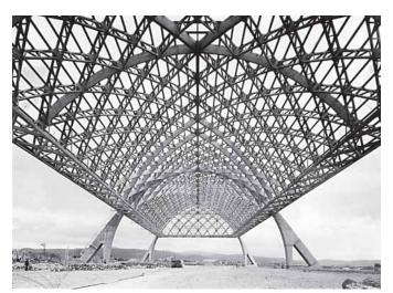
Pier Luigi Nervi's 1936 design of a hangar near Rome, Italy, had a lamella-type shell roof composed of precast reinforced concrete lattice members with only six supporting buttresses. The large ribs were solid, cast-in-place members. *ACI archives. Photo courtesy of Pier Luigi Nervi.*
