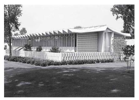
ACI built its first headquarters building in 1957-1958. The principle structural frame was the precast folded plate reinforced concrete roof that cantilevered front and rear from the monolithic corridor walls.
