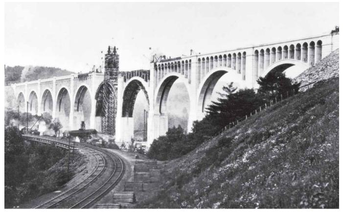
The Tunkhannock Viaduct, Nicholson, PA, completed in 1915, was the largest of its kind ever built of reinforced concrete. The double track viaduct consisted of ten 180 ft (55 m) and two 100 ft (30 m) arches with a total length of 2375 ft (724 m). The structure was 242 ft (74 m) high.
