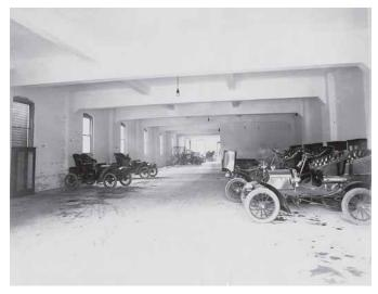
C. A. P. Turner was one of the pioneers in reinforced concrete construction in the U.S. He is credited as one of the inventors of the flat slab system and built the first flat slab, the Bovey-Johnson Building in Minneapolis, MN, on a 14 x 17 ft (4 x 5 m) module in 1906. Turner's system was used in this garage erected in the early 1900s.
