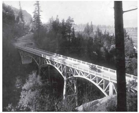
Laturelle Falls Bridge on the Columbia River Highway, built for the Oregon State Highway Commission in 1914, was one of the first concrete bridges in that state. The bridge was considered one of the lightest concrete structures for the load it carried until the advent of prestressing. Engineer-Architect: K. P. Billner. Builder: Harris Construction Co. *ACI archives. Photo courtesy of K. P. Billner.*
