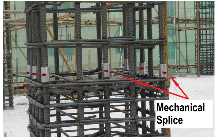
Fig: Bars with Mechanical Splices Source: https://www.structuralguide.com
