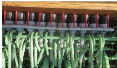
Fig. 1: Examples of reinforcement assemblies that created placement challenges for the contractor: (a) an earthquake-resistant wall; and (b) an anchorage zone for post-tensioning tendons
