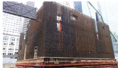
Fig. 1: Examples of reinforcement assemblies that created placement challenges for the contractor: (a) an earthquake-resistant wall; and (b) an anchorage zone for post-tensioning tendons
