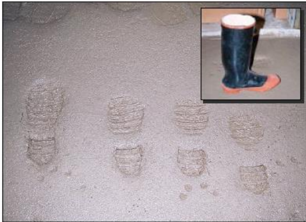
Figure 1. Concrete is generally considered to be ready for floating when finishers leave a ¼-inch-deep footprint in the surface. Using a boot filled with steel shot (inset) to produce footprints, we found that 2½-inch-slump concrete placed on a stone base was ready for floating about 45 minutes earlier than the same concrete placed directly on a vapor retarder.
