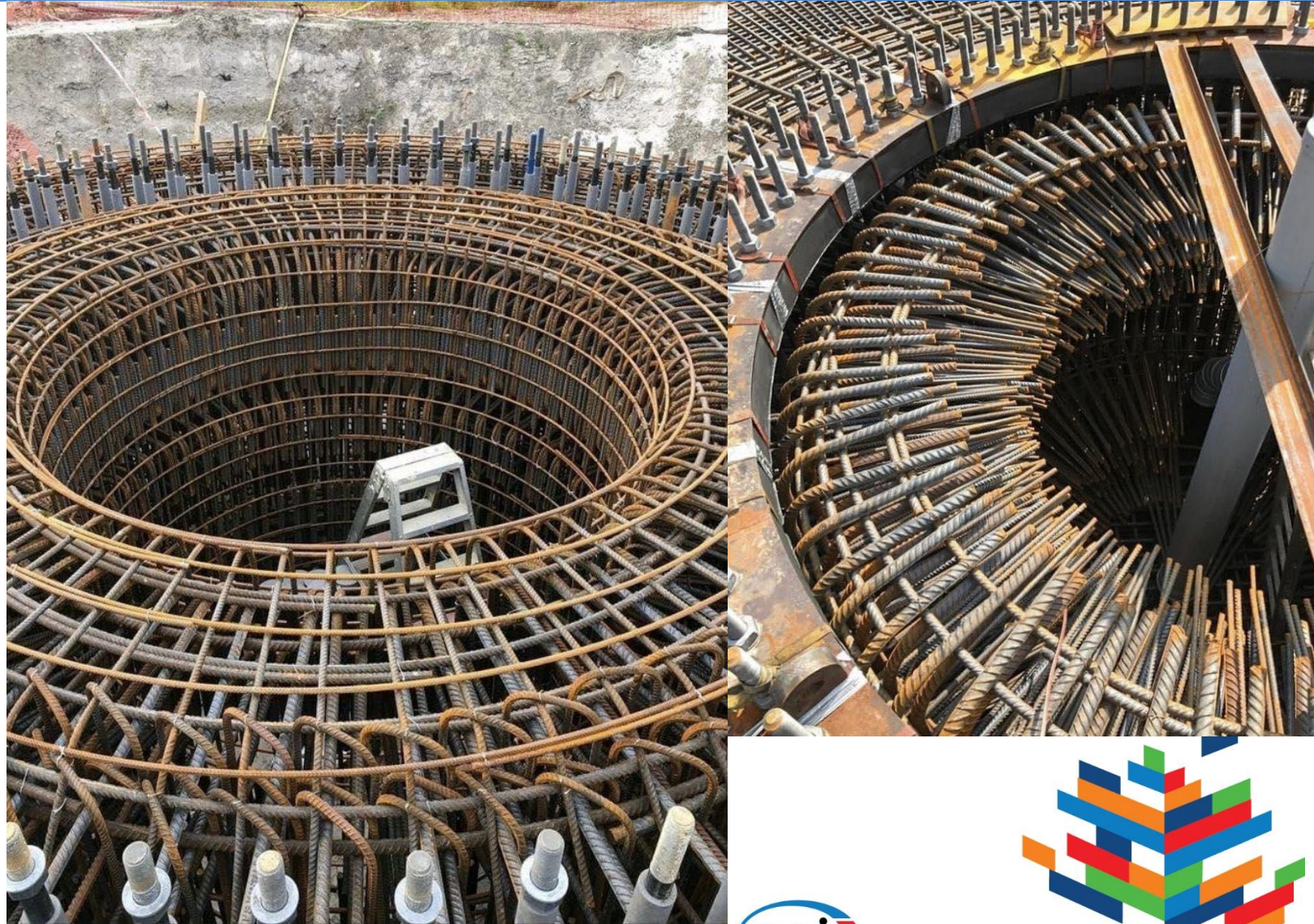
Fig. 1: Examples of reinforcement assemblies that created placement challenges for the contractor: (a) an earthquake-resistant wall; and (b) an anchorage zone for post-tensioning tendons
