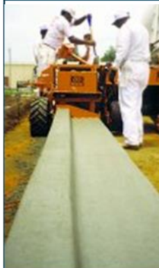
Slipform Concrete
