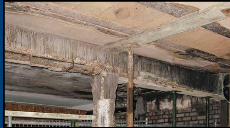
Structural damage to concrete due to spalling
