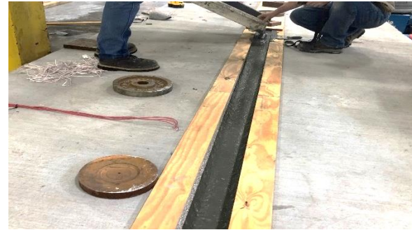
UHPC Joint cast from one end
