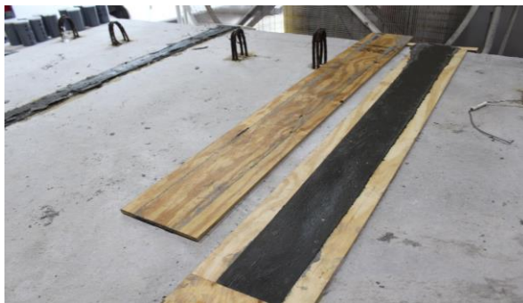
Joint Formwork removal after 24h
