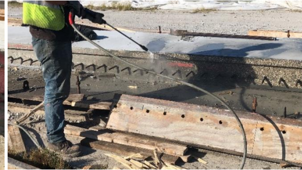
Pressure wash concrete cover
