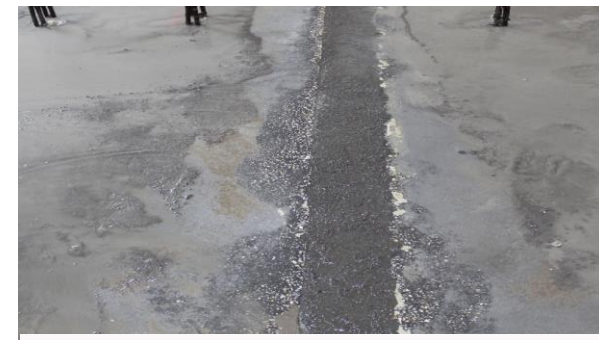
Final joint finish
