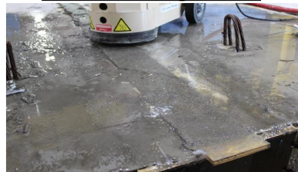
Grinding action of UHPC overpour
