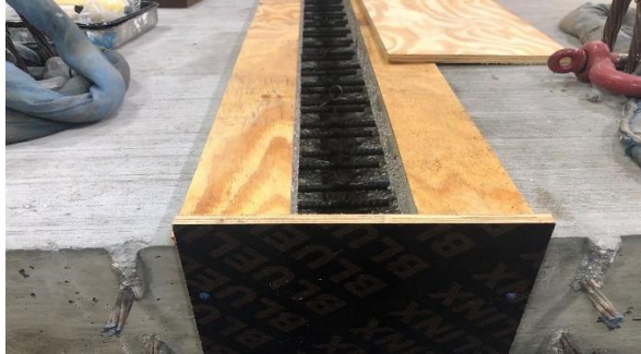
Joint Formwork preparation
