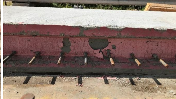
Remove side forms 24h after casting
