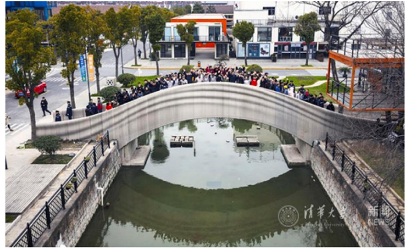
The World's Largest 3D Printed Concrete Bridge is Completed in Shanghai (2021)
