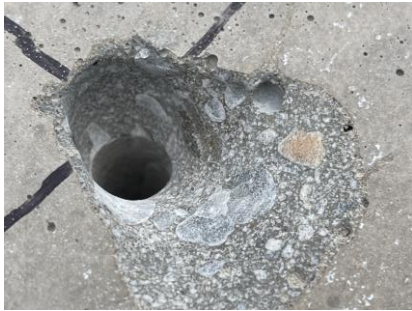
Drilling and chamfering anchor holes
