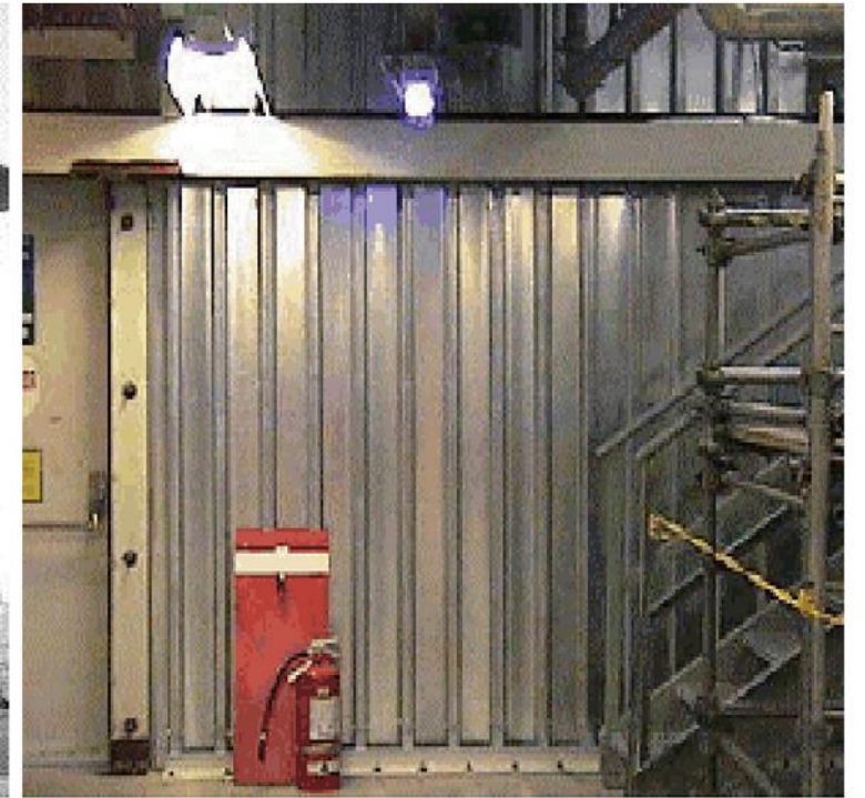
Fig. 10.1.6c—Heavy corrugated steel panel retrofit to CMU panels.
