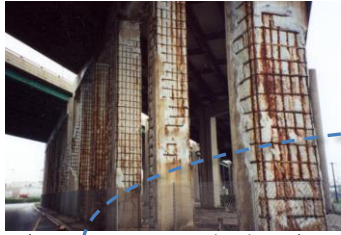
(Vector Corrosion Technologies)
