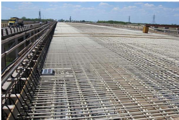
GFRP-reinforced bridge deck
