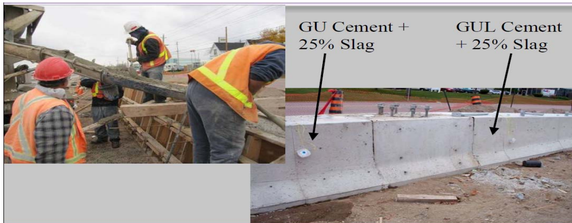
23 m 3 of each mix placed, 30 MPa, 60-100 mm (2.5-4 in.) slump
