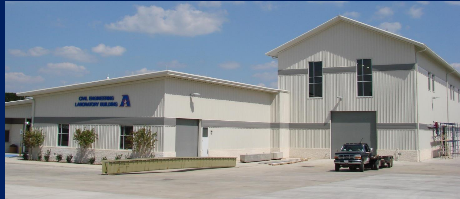
Civil Engineering Laboratory Building
