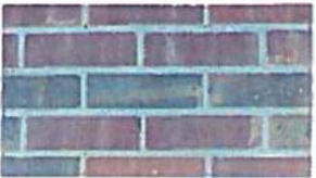
Figure 6. Extruded brick, Type FBS, with a velvet texture
