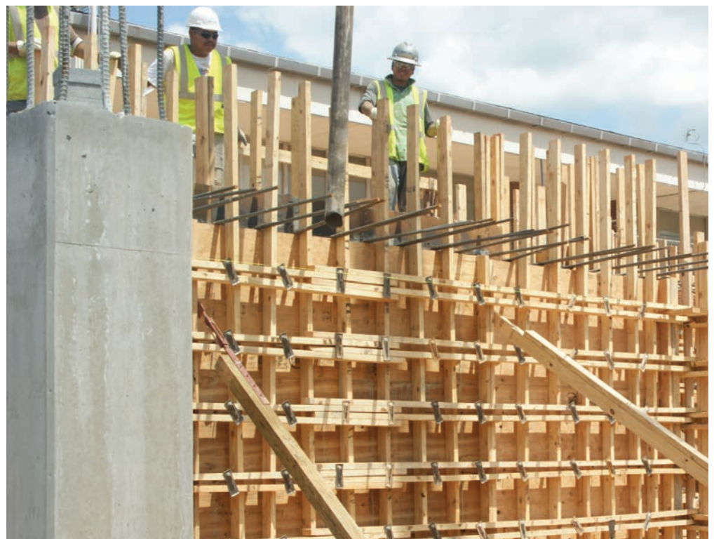
Fig. 1.2: Job-built wall formwork constructed of wood materials
