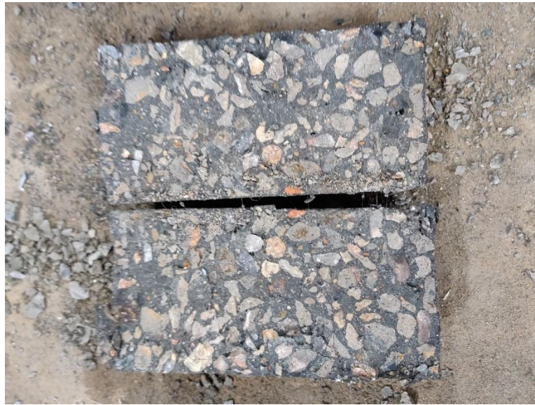
Fig. 3.9: Failure pattern after Tensile Strength Test (28 days)
