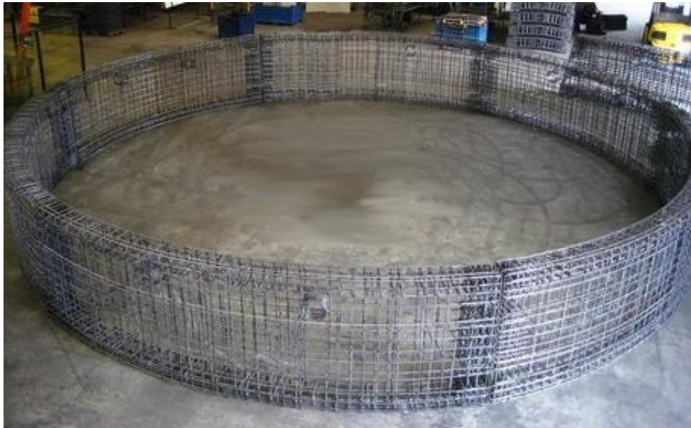
Traditional Steel reinforcement
