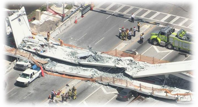
Miami Bridge Failure (2018)
