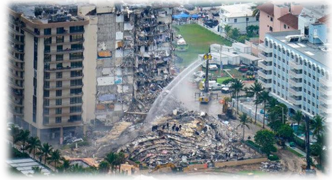
Champlain Towers South Failure (2021)
