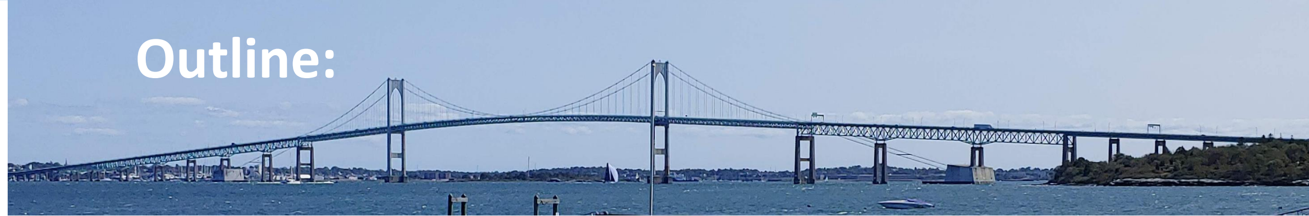
Claiborne Pell Newport Suspension Bridge, RI
