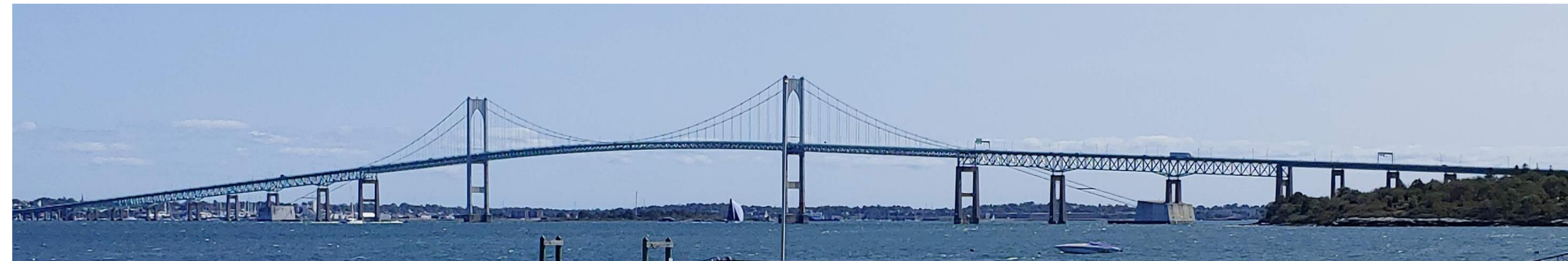
Claiborne Pell Newport Suspension Bridge, RI
