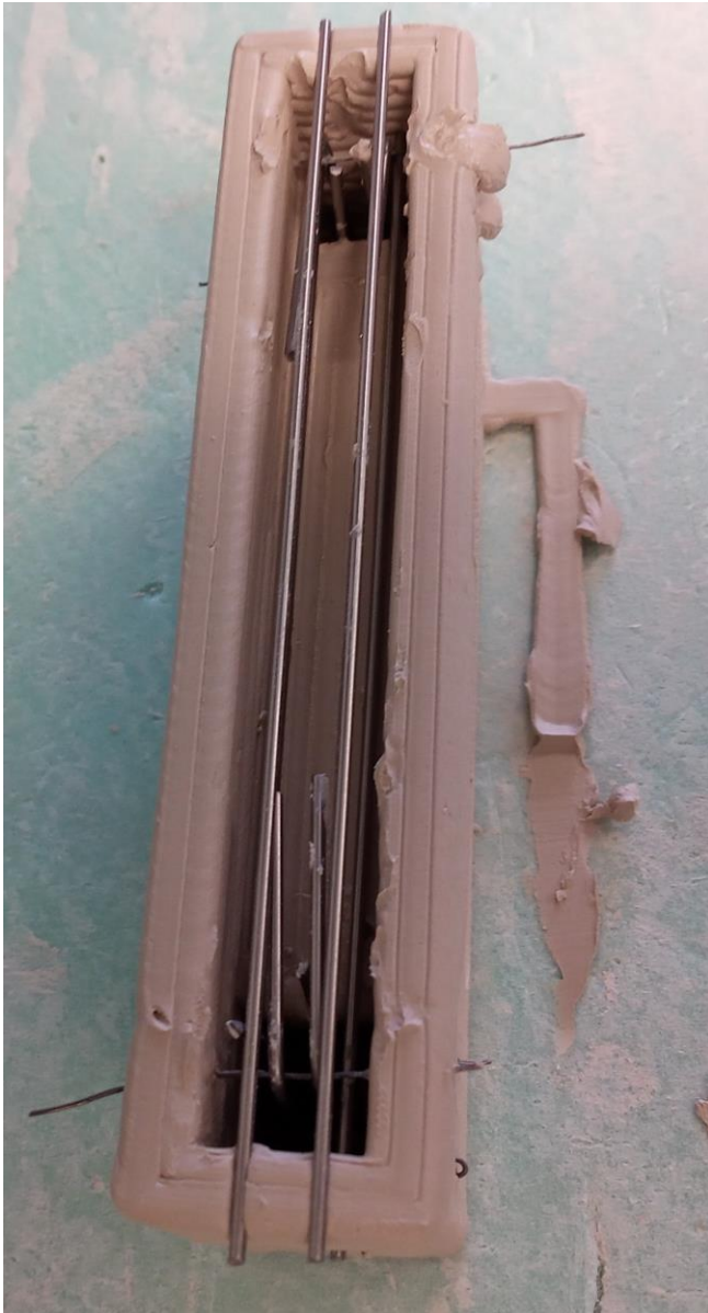
All reinforcement placed
