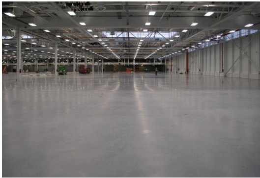
Jointless slabs on ground
