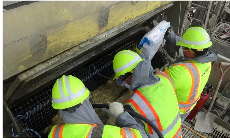
Vibrating the screen for steel fiber addition (2 in. spacing screen)
