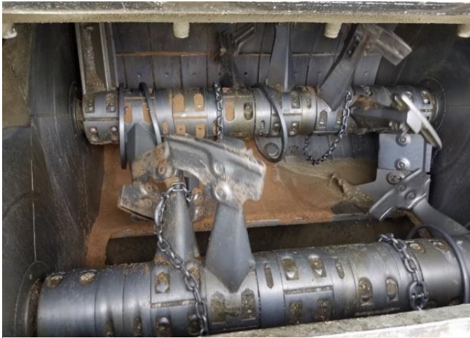
UHPC Mixing using existing twin shaft mixer
