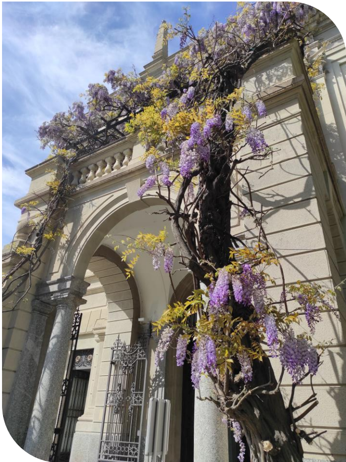
Politecnico di Milano, Building 1 - Rectorate Photo taken by Laura Corti in spring 2022
