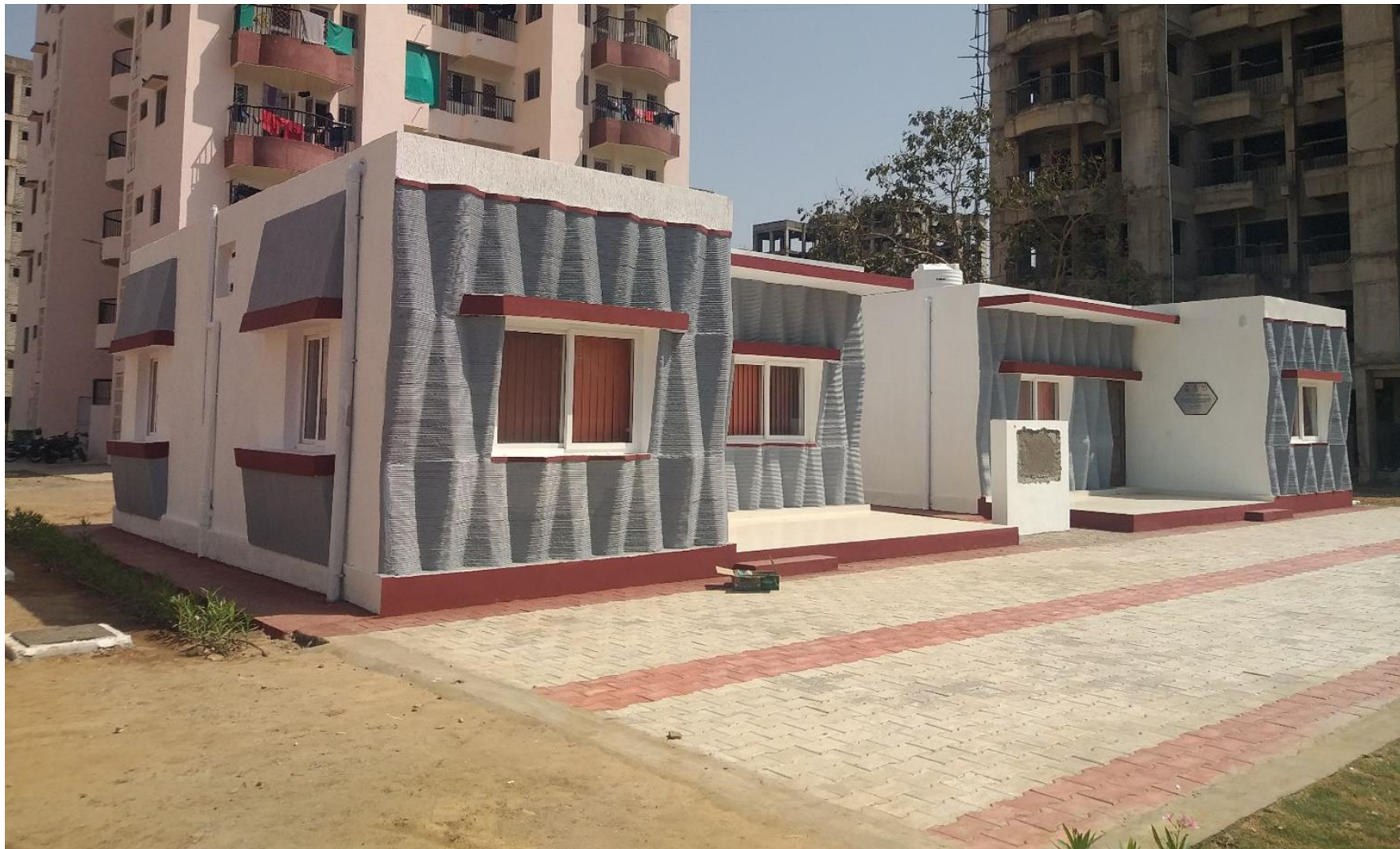
Guest House at Indian Air Force, Chiloda (Gandhinagar)
