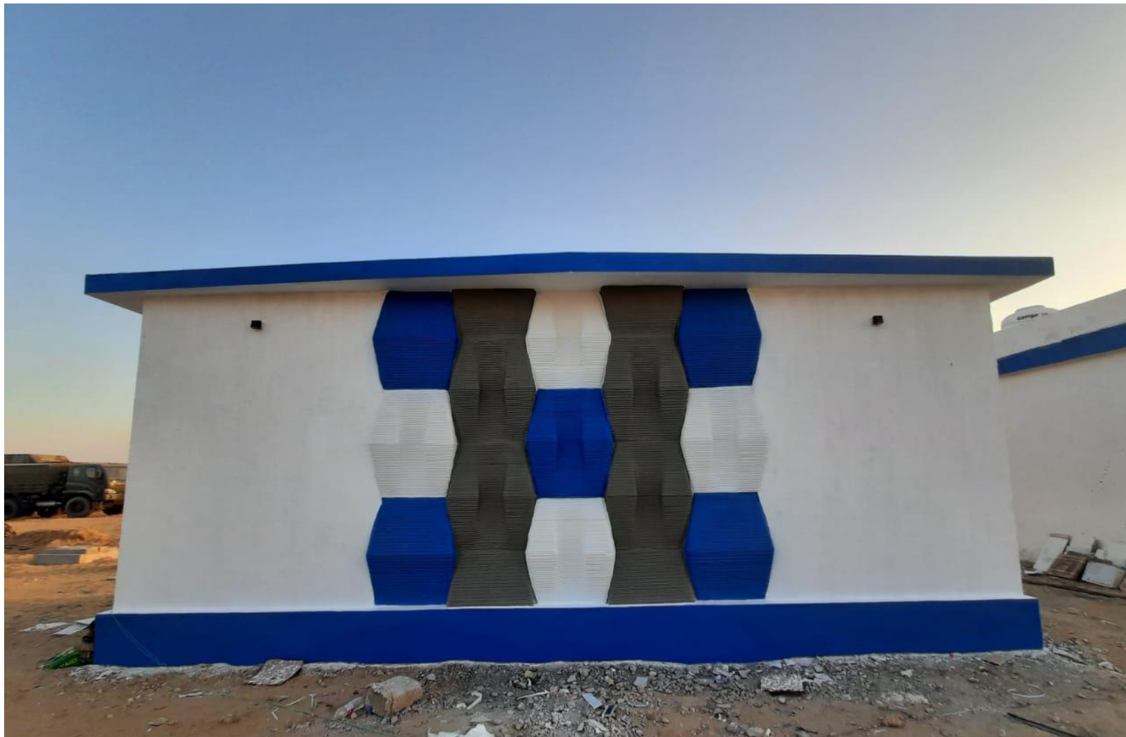
Sanitary blocks at Indian Air Force, Jaisalmer
