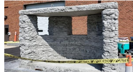
Fighting position – printed walls, roof, foundation
