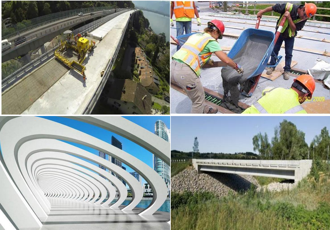
American Mars Hill Bridge, Wapello county, Iowa
