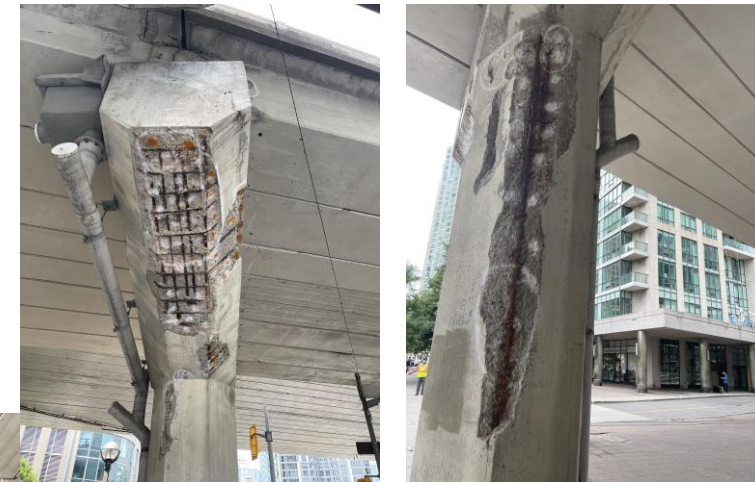
Corrosion in Typical RC Bridge Piers (Mohammed Al-Ani, 2015)
