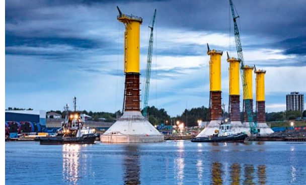
Offshore wind turbine concrete fixed base foundations
