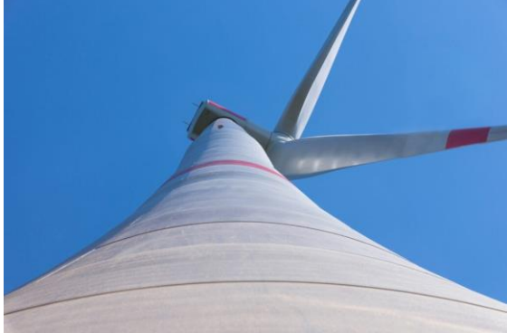
Onshore wind turbine concrete towers
