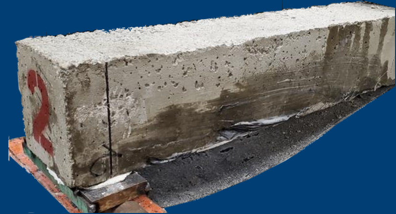
Beam 1 after testing (b) Beam2 after testing – Intermediate crack debonding failure mode
